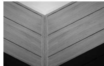
Figure 13, Image at inside corner with two J-Mold Trims
