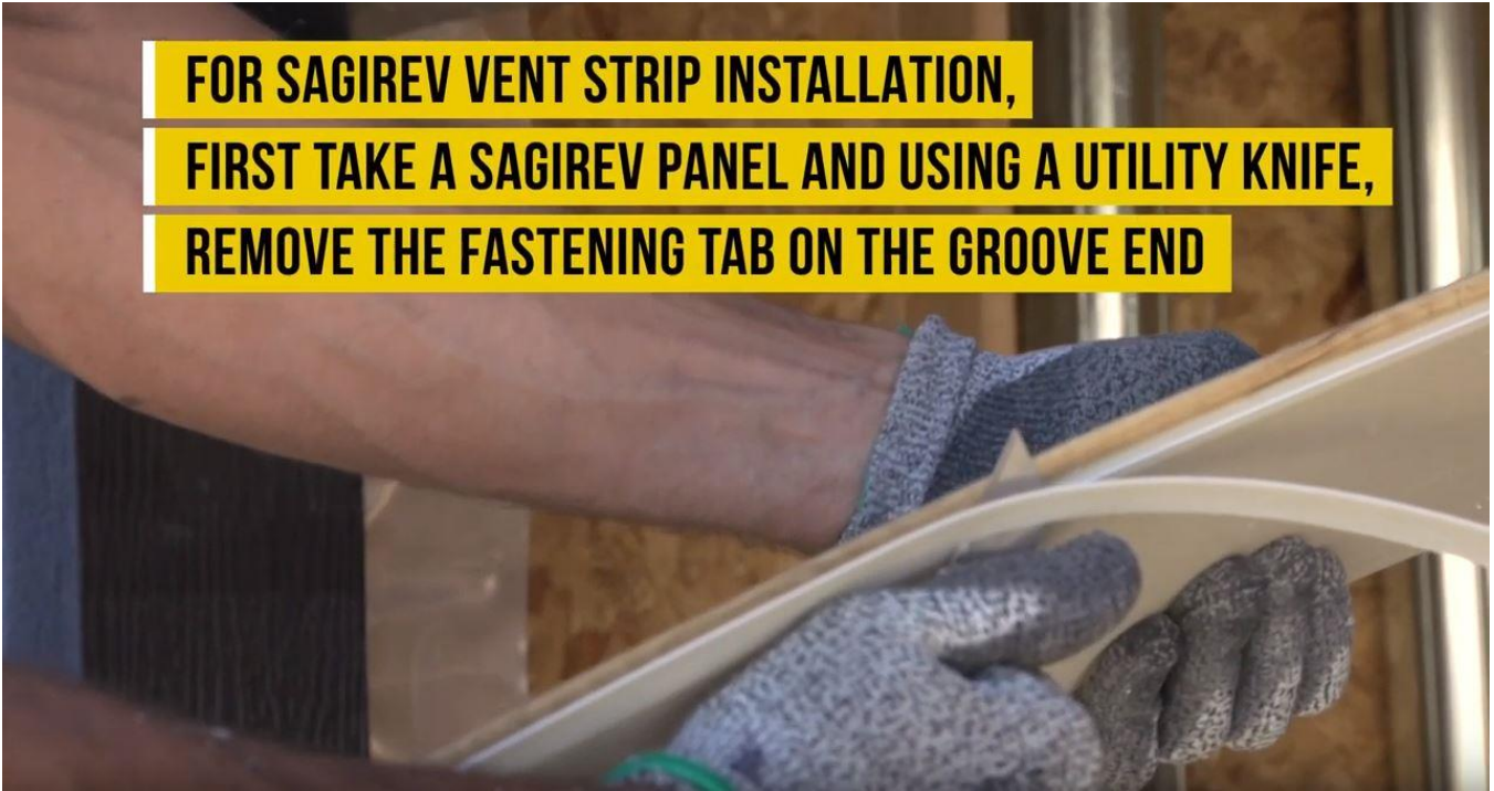
Figure 21, Remove nailing flange
