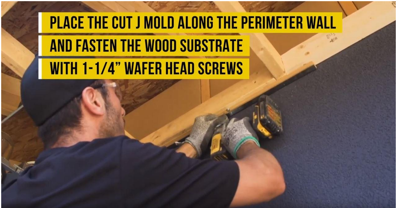
Figure 18, J Mold Trim at soffit, prior to installing soffit boards
