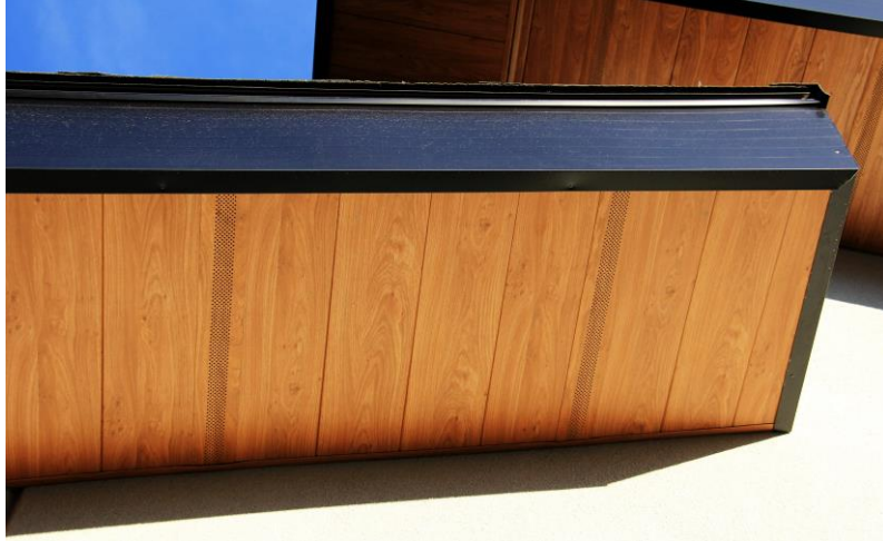
Figure 16, Soffit with SAGIREV Vent Strips, perpendicular application
