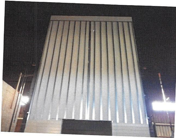
Figure 4. Wall System Under Construction.
